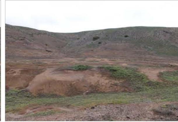
Photo 108: Section 5 Water Pipeline
