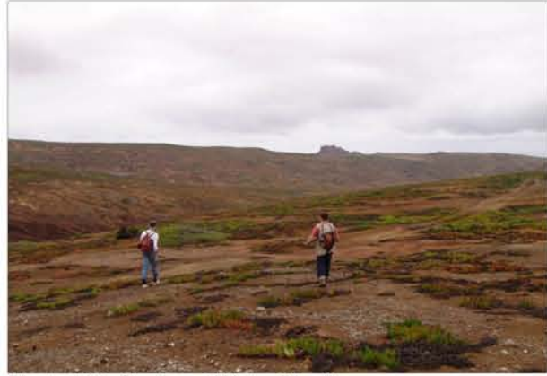
Photo 105: Section 4 Water Pipeline
