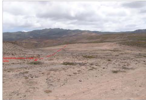
Photo 110: Section 7 Water Pipeline Location
